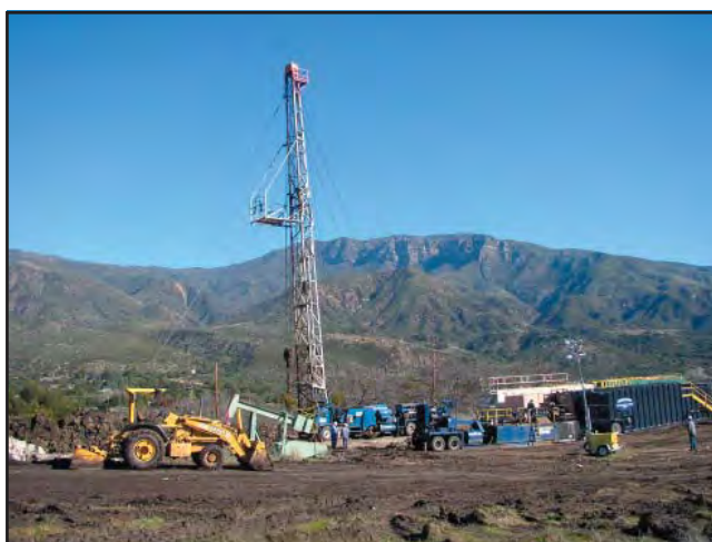
Photo 2. Key Energy Services California Inc. rig during abandonment operations on well "Ojai" 36. The Topa Topa Mountains are in the background. Photo by D. Kahler.
